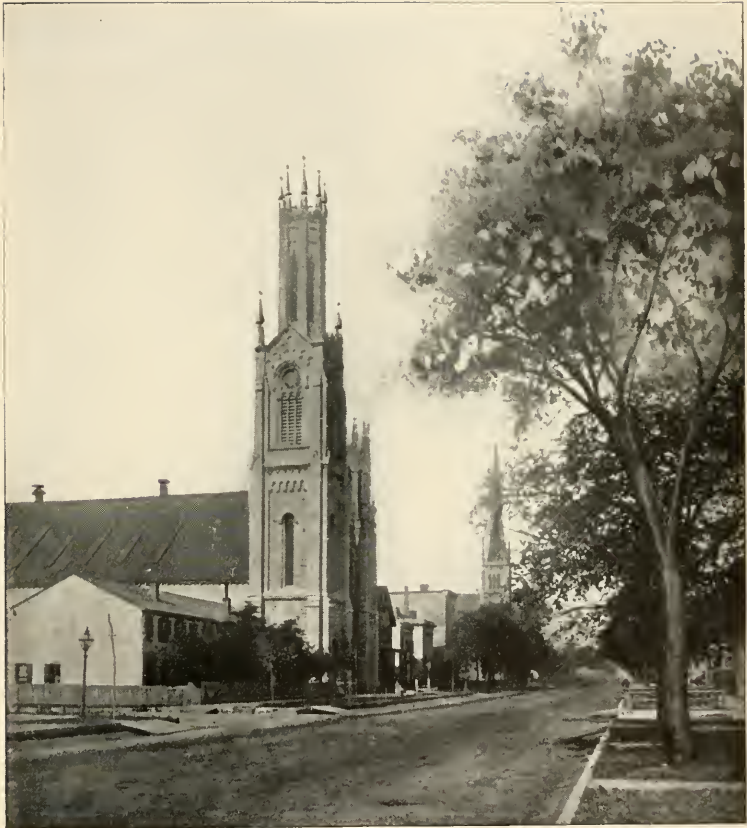
THE FIRST PRESBYTERIAN CHURCH, 1866—WABASH AVENUE NEAR CONGRESS STREET.
